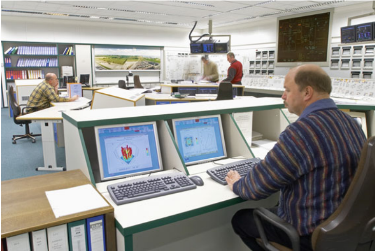
Fig. 2.2 NPP control room in Germany (Photo by GfS/KSG, Essen, Germany), because the room is windowless, the control room teams have hung up a poster with the outside view (in the back). Files with standard operating procedures on the shelves
