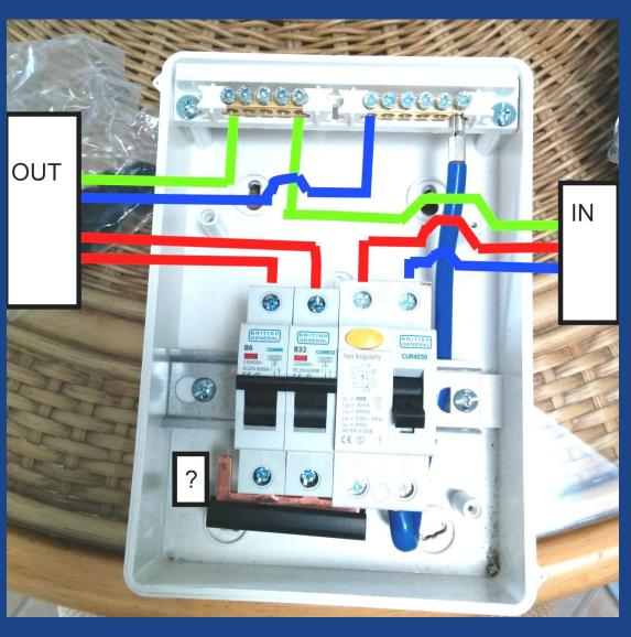
It is important that any holes made for cable entry are no larger than they need be. The cable installation entry method shall, as far as is reasonably practicable, maintain the fire containment of the enclosure.
