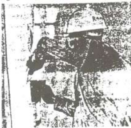
Figure 3-3. Securing lap and butt joints with staples
