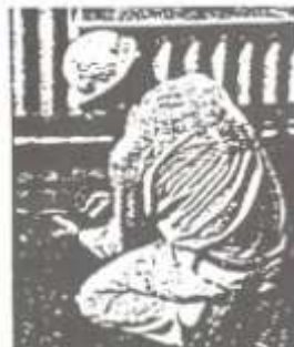
Figure 3-6. Installing cellular rubber insulation
