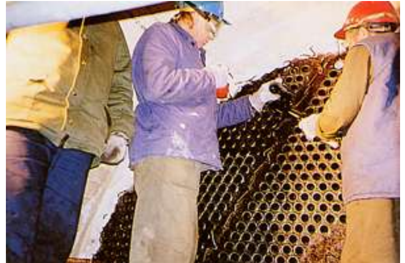
Weld preparation of heat exchanger tube sheet prior to welding
