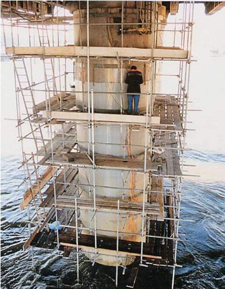
Cracked columns on Charing Cross Rail Bridge. Fractures extended top to bottom for 10 metres
