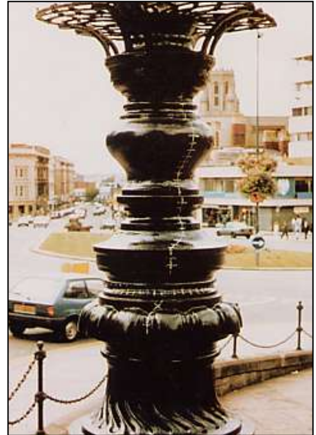
Cracked architectural flagpole
