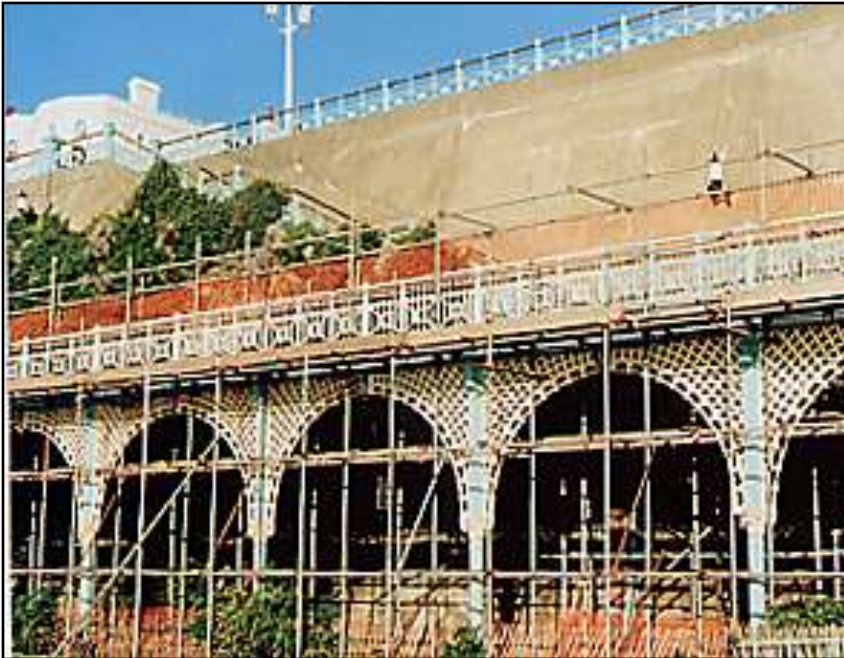
Spandril and railing repairs to Madeira Drive - Brighton
