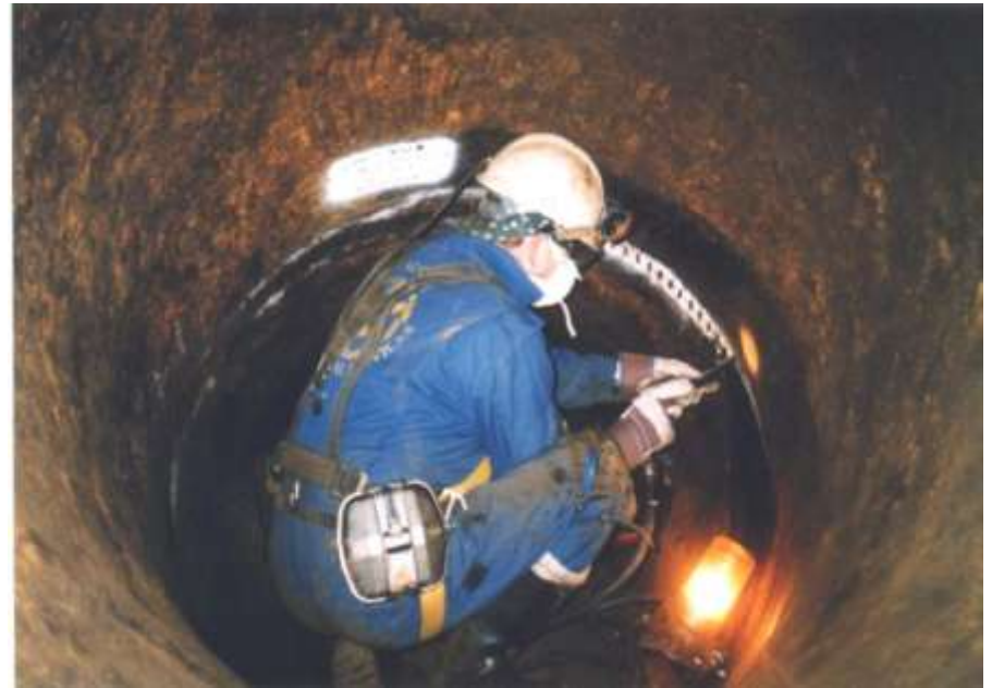
Metalock repair to severe cracking in 48 inch diameter cast-iron water main
