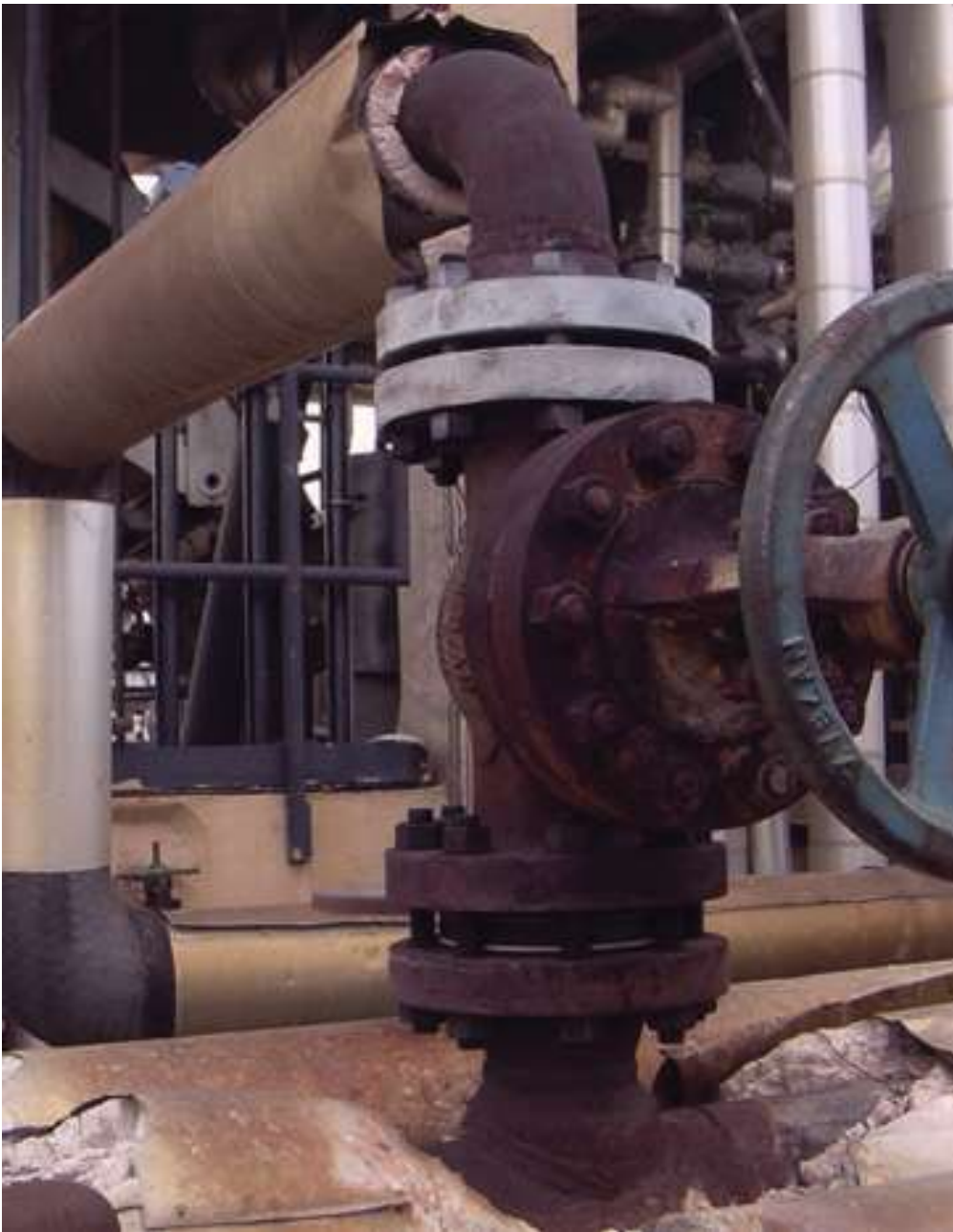
Missing and damaged insulation and jacketing on a valve and connecting piping.
