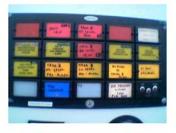
Whenever a process alarm has activated, it must be acknowledged (and silenced) by first pressing the *accept* button on the alarm panel. The *reset* button must then be pressed to see if the alarm condition has cleared or cancelled. The system is so designed so that once initiated these alarms *will not self cancel*, therefore requiring process operator attention.
