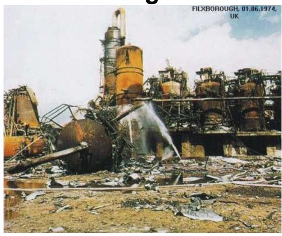
Two months prior to the explosion, a crack was discovered in the number 5 reactor. It was decided to install a temporary 50 cm (20 inch) diameter pipe to bypass the leaking reactor to allow continued operation of the plant while repairs were made.
