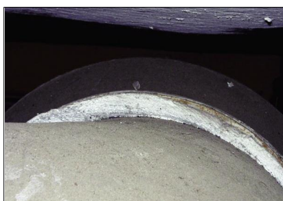
Joint packing on a flue
